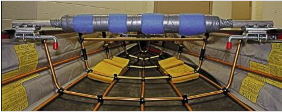
The new yoke installed
